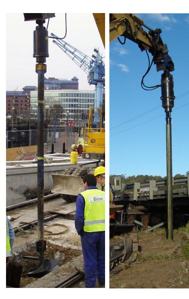
The New Diggalign Inclinometer was developed for contractors where accuracy is key. Ideal for drilling, screw piling and core barrelling applications. Designed to show the operator when the top of the pylon/pile/auger is off plumb, helps to maintain accuracy through out the installation.
